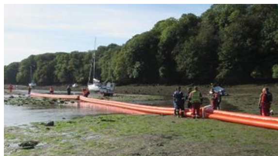
▲ Valero Pembroke Refinery participates in an oil-spill exercise to deploy booms to protect an environmentally sensitive salt marsh. The booms are anchored and chained, and designed to divert oil to an area where it can be recovered.
