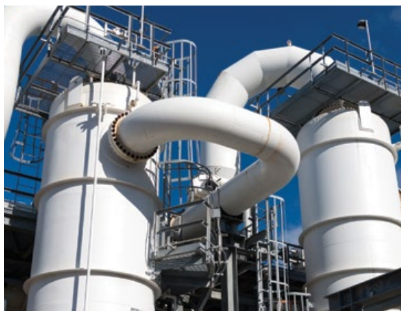
▲ Flare-gas recovery systems, like this one at the Bill Greehey refineries, capture and recycle gases.
