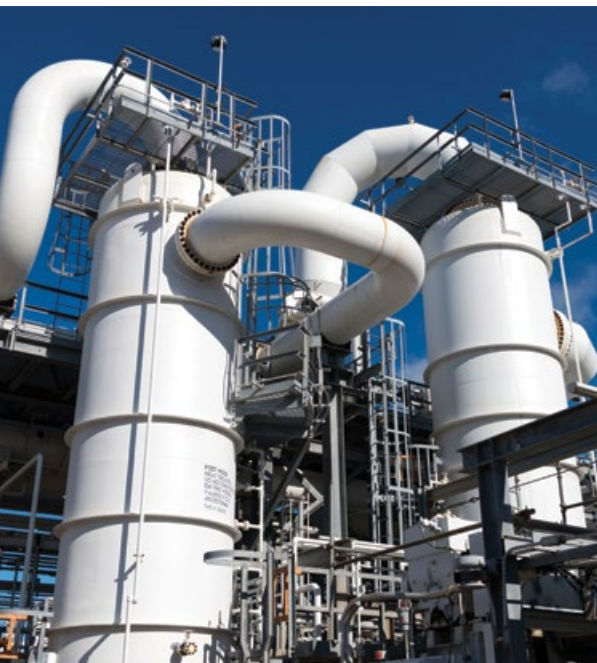
The flare-gas recovery unit at the Corpus Christi West refinery is part of Valero's companywide flaring reduction initiative.
