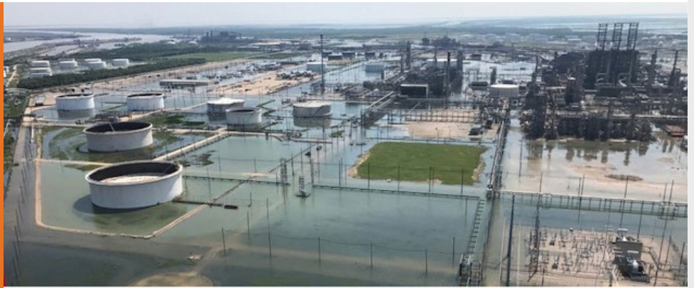
The Port Arthur refinery sits in flood waters in the aftermath of Hurricane Harvey. Preparations ahead of the storm, and quick action during, allowed the refinery to begin restart within two weeks.
