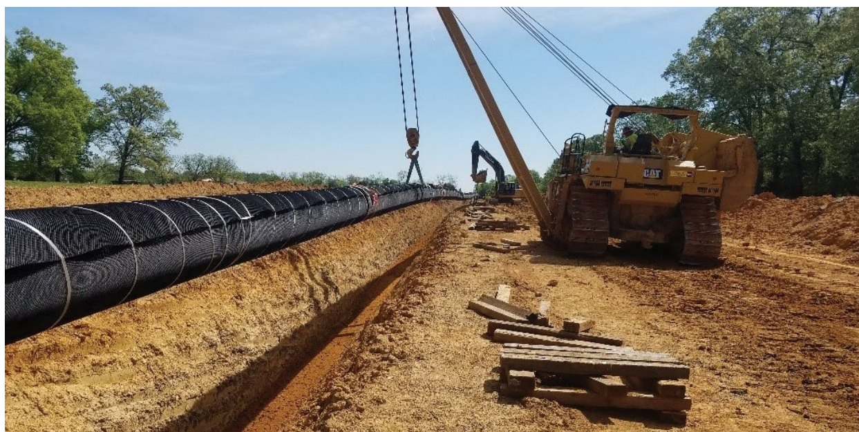
Valero completes construction of the Diamond Pipeline, in partnership with Plains All-American. U.S. Department of Transportation statistics show that underground pipelines are one of the safest modes of transporting crude oil.
