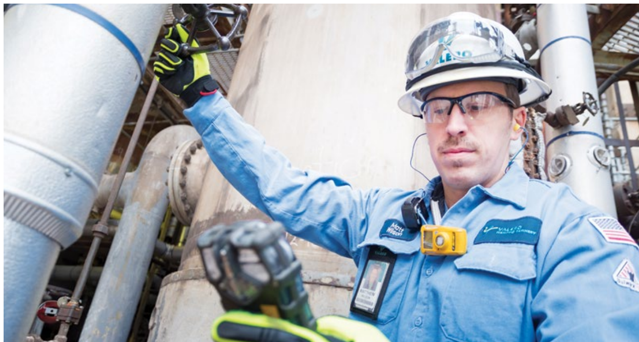
Matt Wilson, Assistant Operator, inspects piping at the Memphis refinery.
